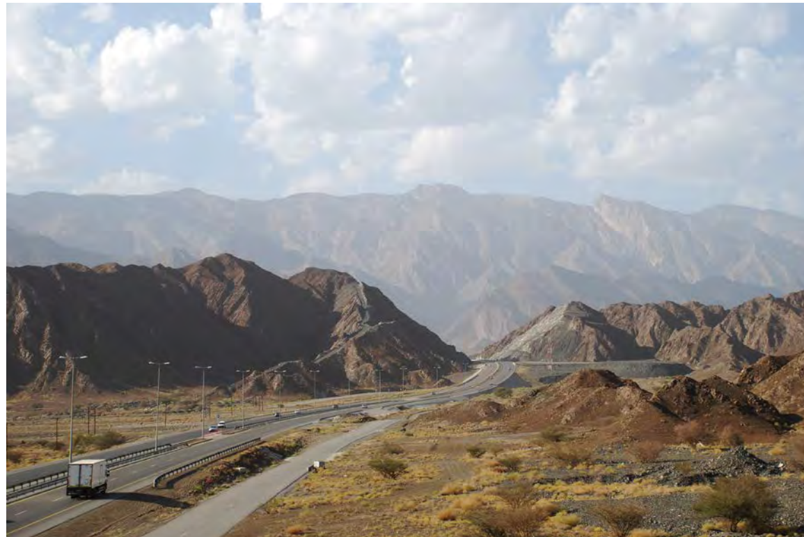
Highway Sohar to Al Ain (UAE), Studio Basel Preparation Trip 2012
