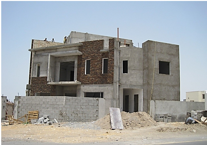
Picture 23: Villa-model is characterized by large openings and energy-inefficient building materials
