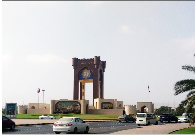
Picture 31: Burj Al Sahwah Roundabout
