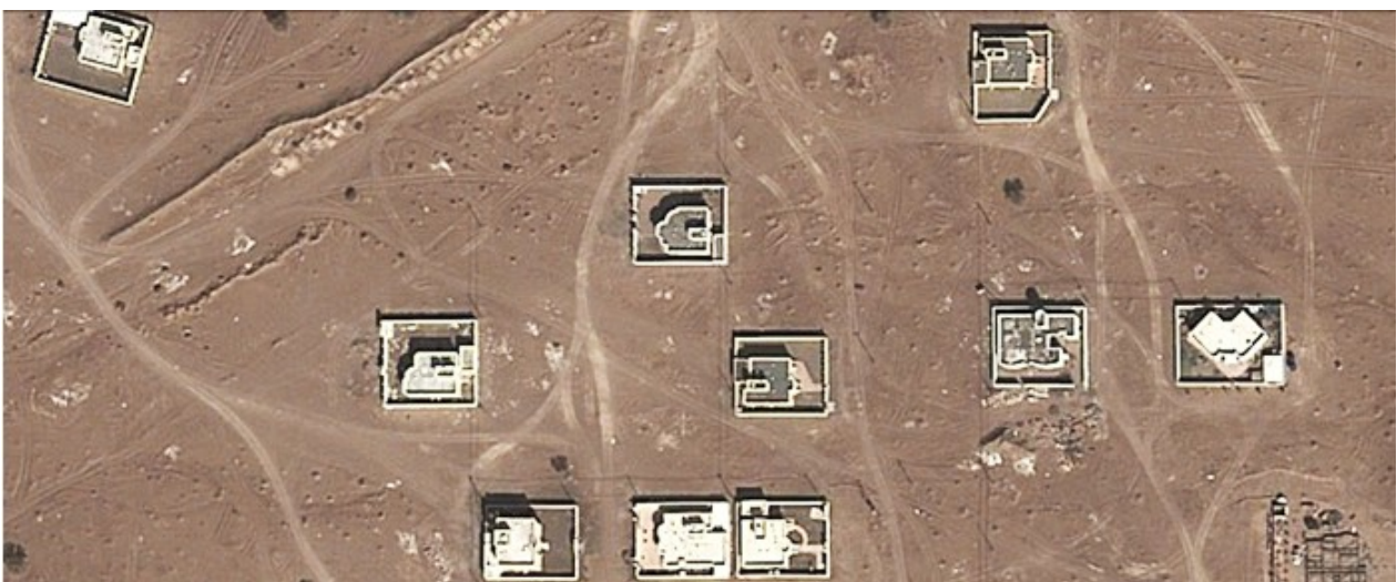
Picture 43: Low-density built form contributes to extreme consumption of energy.
